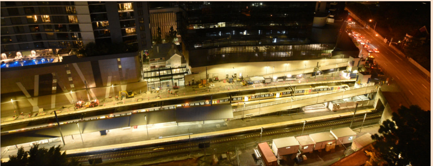
Night shift on the South Bank station upgrade.
