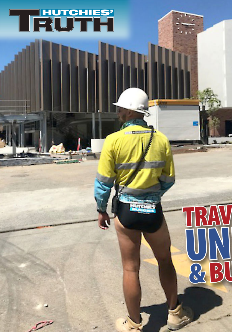
Site apprentice on the West End State School expansion project, Jaime Wiki, stripped down for Fancy Friday.
