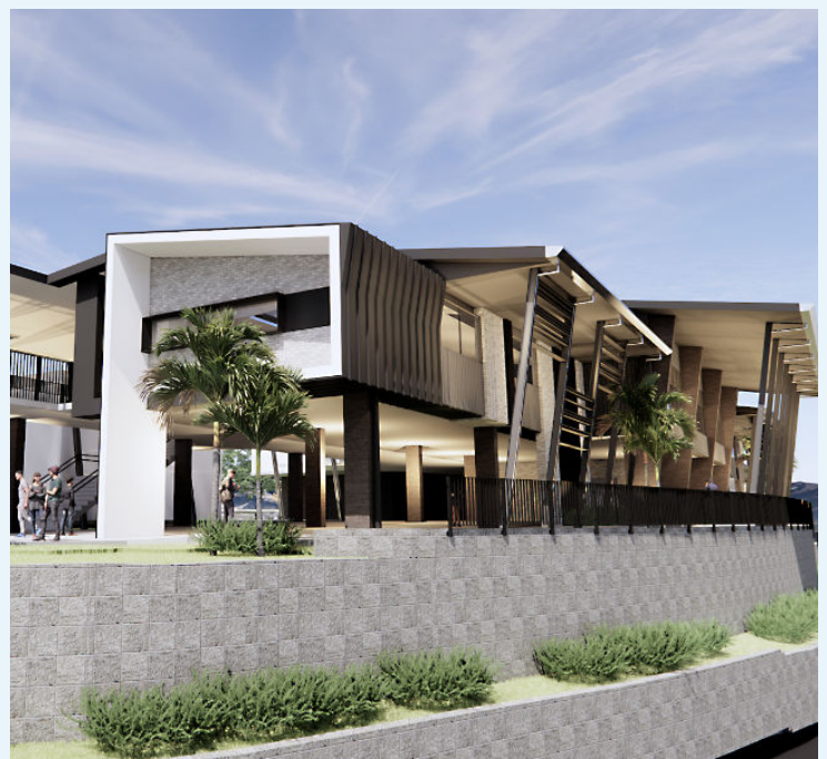
A new junior secondary precinct under construction within the Pacific Pines State High School will cater for an extra 650 students.
